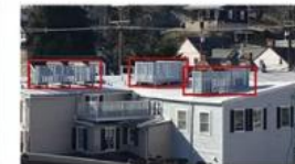
Relocate HVAC units to rooftops or upper porches to protect from flooding and also to be hidden from public view
